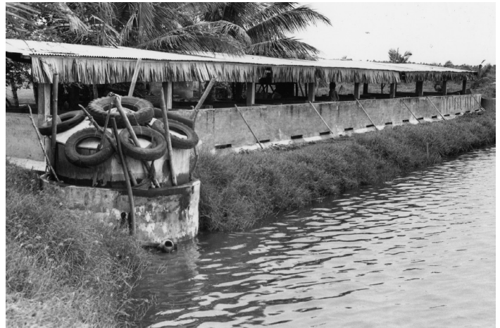
Manure, flushed from hog pens to silo (tires on top), produces biogas for domestic use. Effluent waste from the silo then flows into a pond to enrich waters for growing fish. Fish processing wastes are fed to hogs, Tigbauan Iloilo, Philippines.
